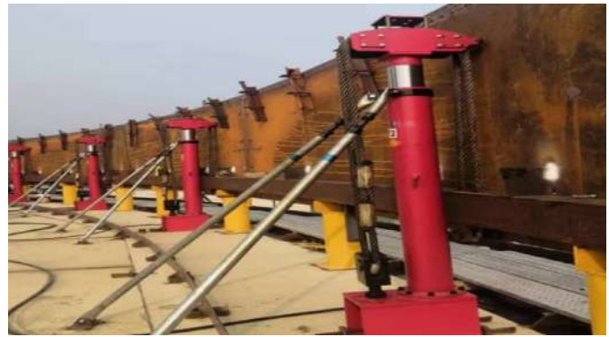
Hydraulic Jack For Tank Lifting
