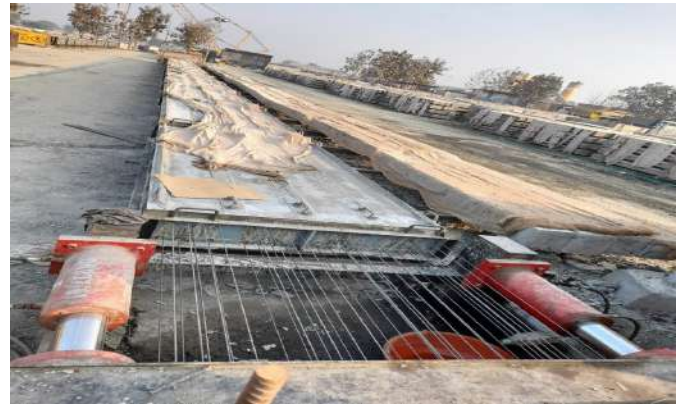
Hydraulic Jack Wire Stressing
